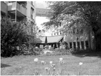
The service house Blandaren in Linköping
